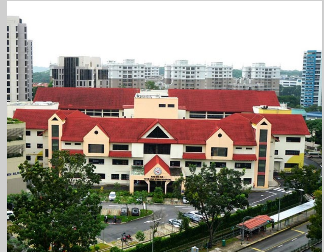
Picture shows the existing building and roof tiles will be recycled and reuse it as building construction aggregates and pavements to the public spaces.
