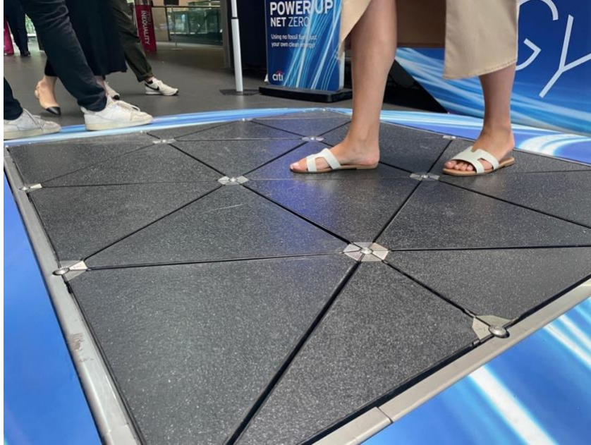
Pavegen Harvesting energy flooring systems located at Citibank, London
