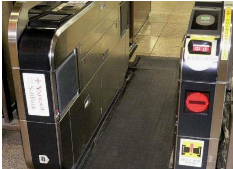
Soundpower's Generating Floor Mats located at Shibuya Station, Japan
