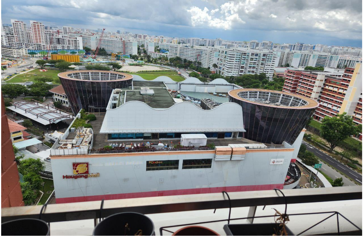
Figure 4: Rooftop View of Hougang Mall
