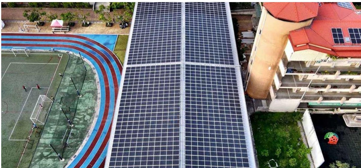
Figure 16 Solar Panel Roofs at Taiwan New Taipei City's basketball court
