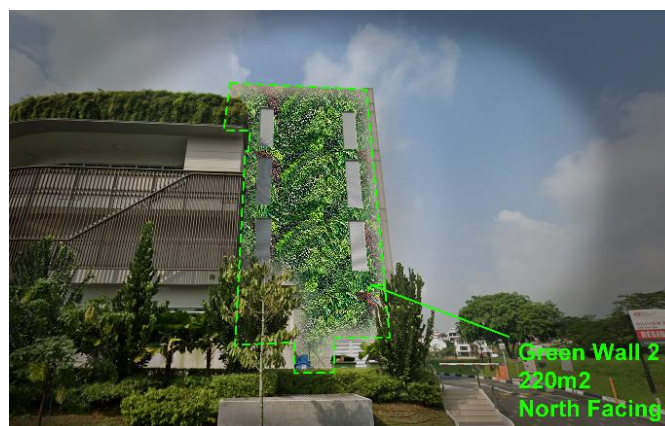
Figure 35 Location of LLC Panel, Green Wall 2
