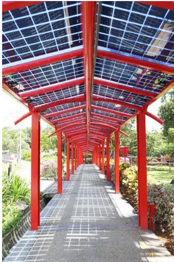
Figure 42: Singapore Discovery Centre Sheltered Walkway Solar Panel
