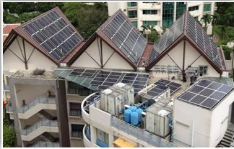
Figure 43: Solar Panels at Homes@Hongshan
