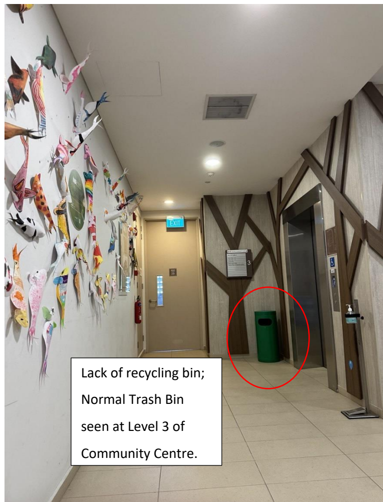
Figure 26: Bin at Level 3 of Hillview Community Centre
